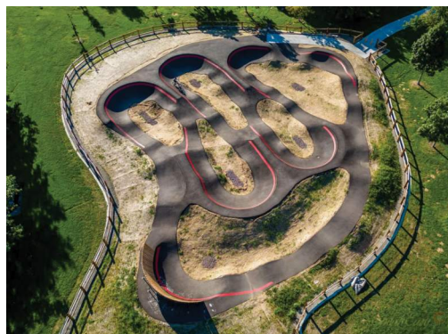
Montebello Pump Track Denver, CO (~14,000 SF)
